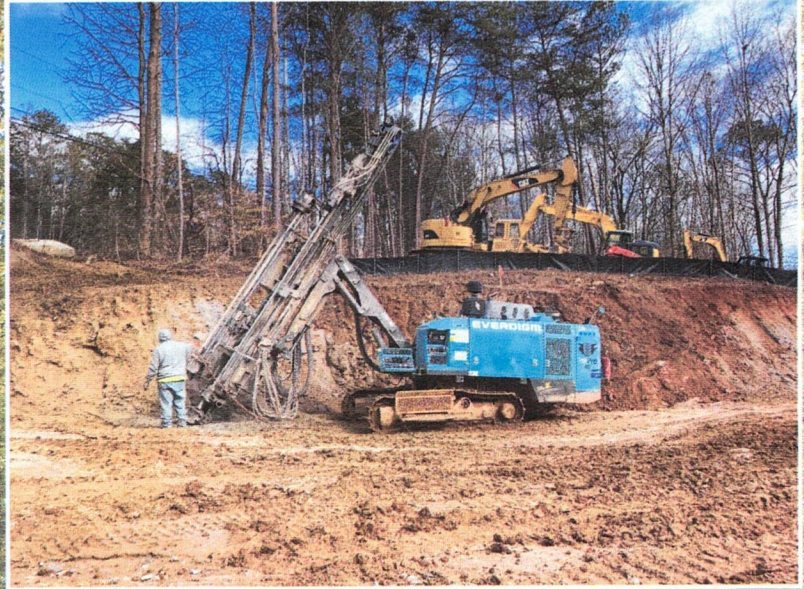
Dawson Forest Road Lift Station & Sanitary Sewer Project Work
